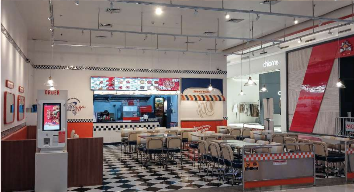
○ Pekerjaan Fitting Out Gopizza Mall Of Indonesia
